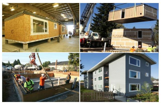
Modular housing can be assembled in the factory while the site preparation work is being completed. Once the modular units are delivered to the site, the buildings go up guickly.
